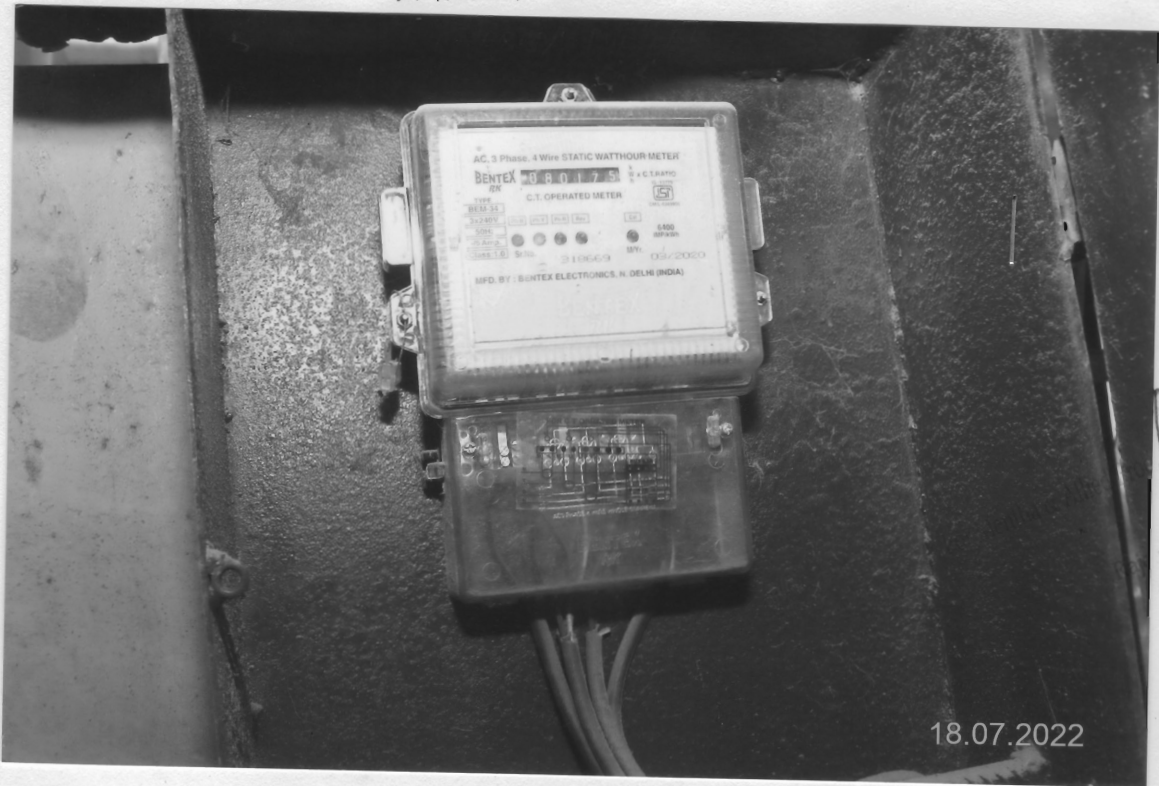
TFH 15 LAC + STEAM BOILER ENERGY METER
